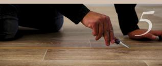
Insert the end of the nozzle in the joint and work backwards, slowly injecting the fluid until it overflows at the surface on the paper adhesive tape.
