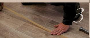
Apply masking tape along the joint.
